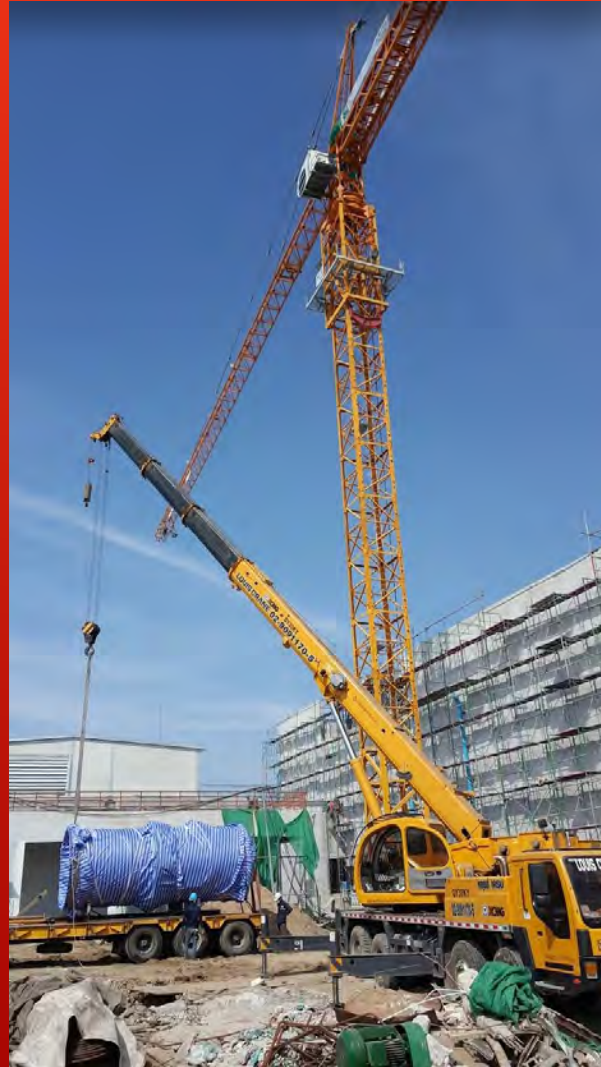
Move Silo By Tower Crane
