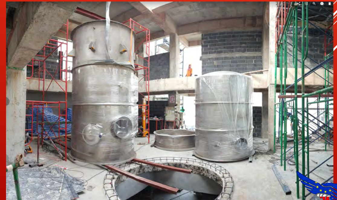
Silo Installation Work
