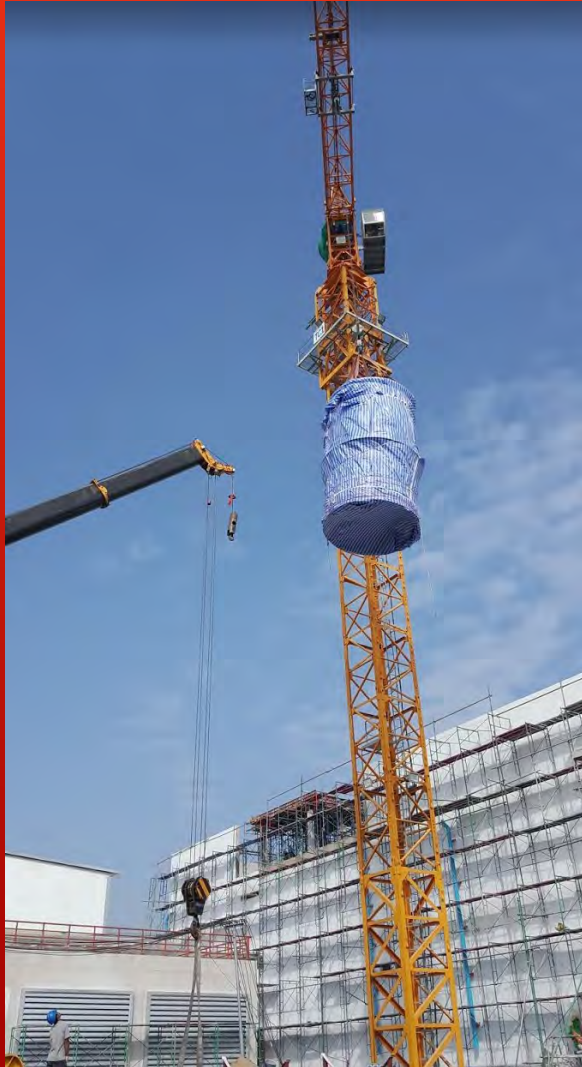
Move Silo By Tower Crane
